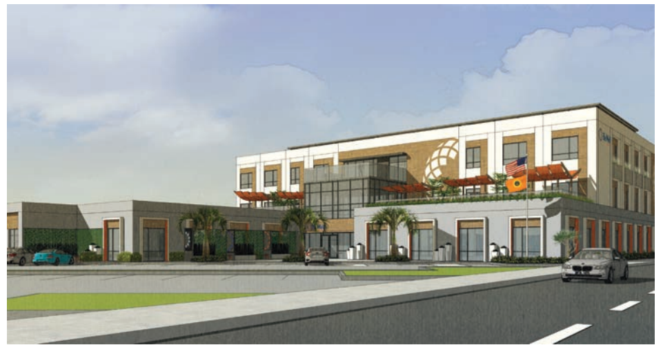
$40M estimated cost for Orange facility; 10K visits per year expected
